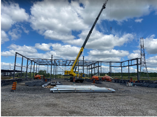
Figure 2. The selected project in this study
